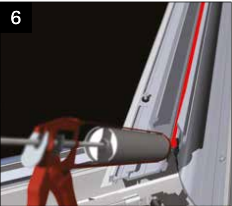
Now run a continuous bead of suitable silicone down the entire length of the aluminium valley profile, at the point of the hinged connector in the centre.
