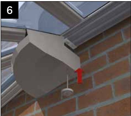
Screw threaded rose cover into the fixing 'point' mounted on the aluminium hub end.
