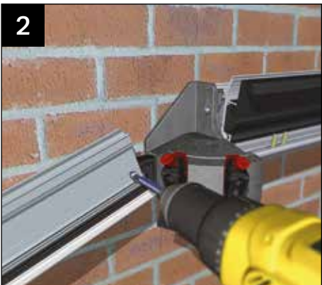
Prior to attaching the starter bar to the mounted starter bar bracket, remove the M6 tapite screw. Locate the bar on to the bracket and on to the single bolt placed in the eaves beam, re-insert the screw.
