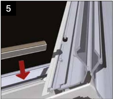
Cut and re-fit the glazing support trim, where the valley meets the eaves beam.
