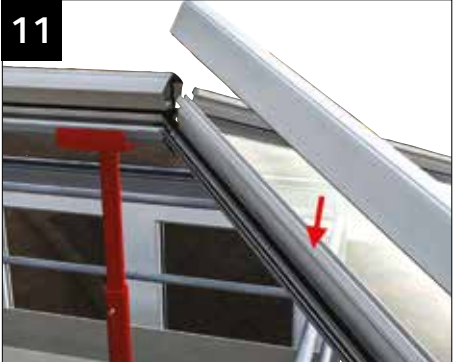
Work your way around the roof and fit glazing bar top caps.
