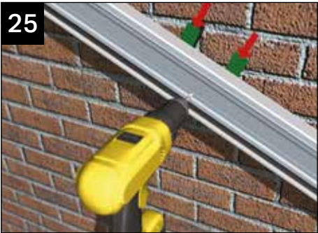
Drill the starter bars/masonry within 200mm of the ridge and eaves beam plus at least one more equidistant between the two. Pack out to support the starter bar behind each fixing before fitting the correct masonry anchor. If necessary pack behind the ridge too with aluminium shims.
