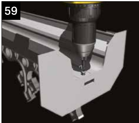
Screw the flashing trim to the ridge top cap through the screw port. Use a 4.2mm x 13mm self drilling screw (not supplied).
