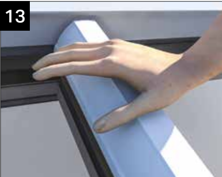
Using the heel of your hand, push down on the top cap to engage the clips, working from ridge to eaves. Ensure the rubber gaskets are full compressed for a watertight seal. NOTE: on longer bars it may be necessary to use a soft mallet and timber block
