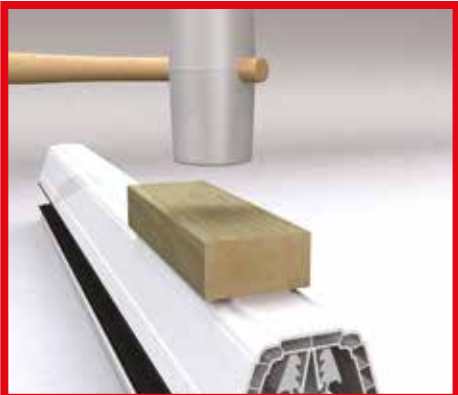
Knock the glazing bar top cappings on with a Deadblow hammer. Greater care is needed in cold weather. Keep all trims wrapped until they are needed. Once again each capping is numbered according to its position in the roof.
